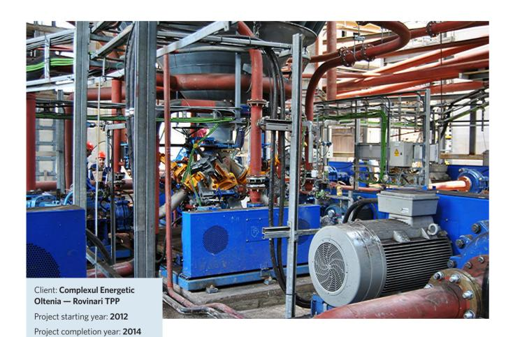
In order to provide an appropriate operation managed by the DCS, it was required to replace an important number of valves, provided with DCS-compatible actuators and safety valves for the operation of the power unit.
